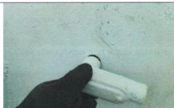
Obsolete conduit entering tank roof is loose
