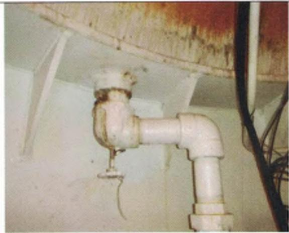
Mud valve under the inverted cone
