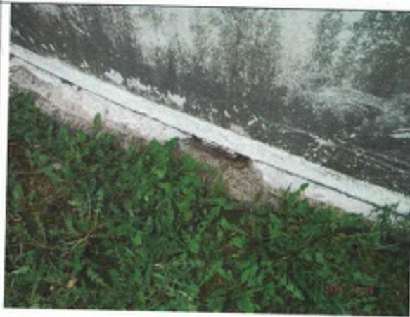
Spalling of foundation
