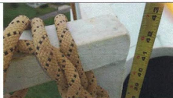
Roof handrail is 42" in height
