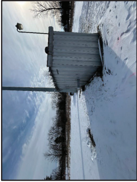
Photograph 1 - Allendale Avenue Well House (LW1), Looking East
