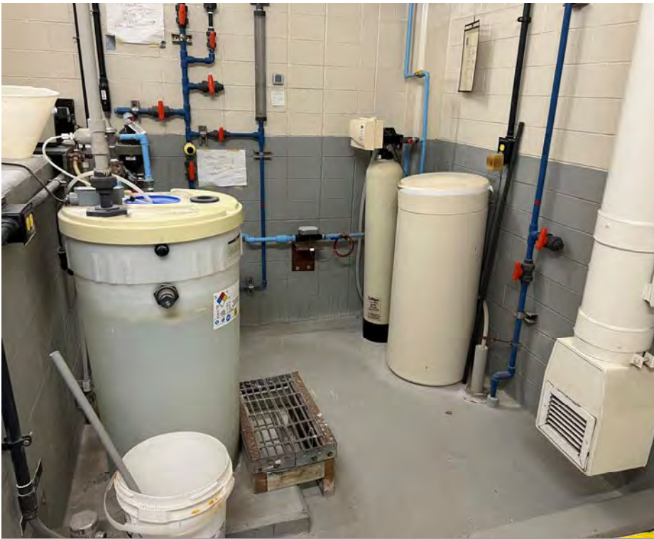
Upflow saturator and fluoride feed equipment
