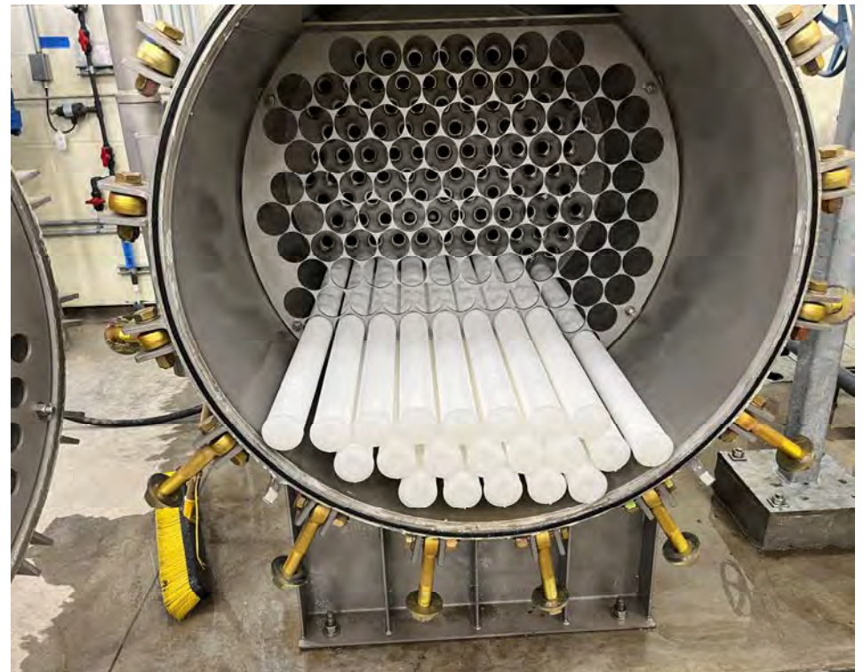
Harrison (OH) WTP – Cartridges and Filter Vessel
