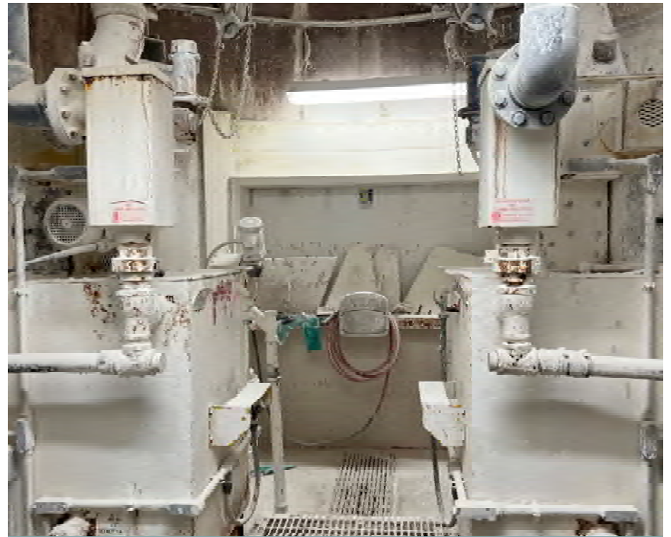
Continuous Lime Slurry Slakers
