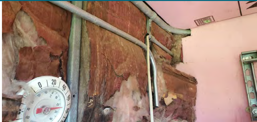
Local Well 1 Interior Insulation
