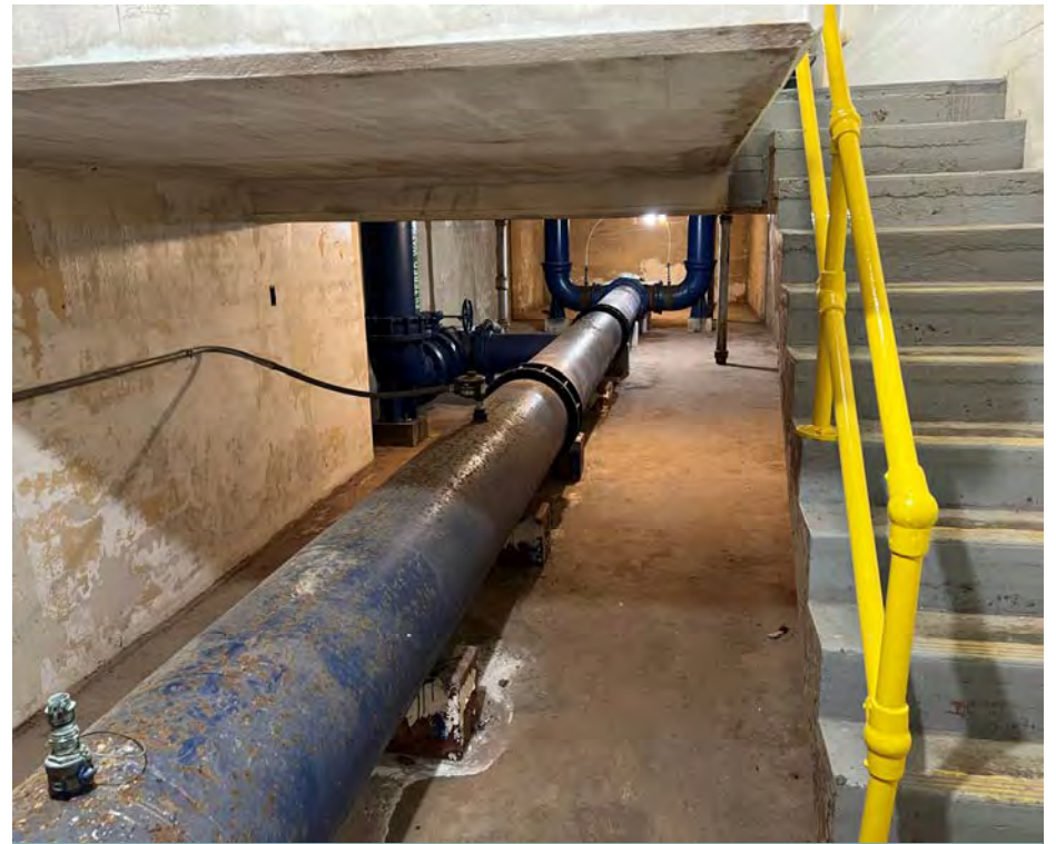
Filter Effluent Piping to Underground Storage Tank
