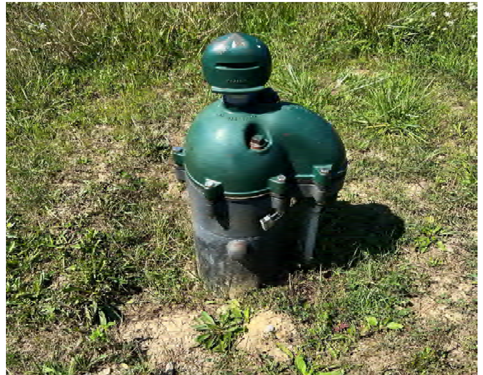
Hintz Well Pump Pitless Adapter
