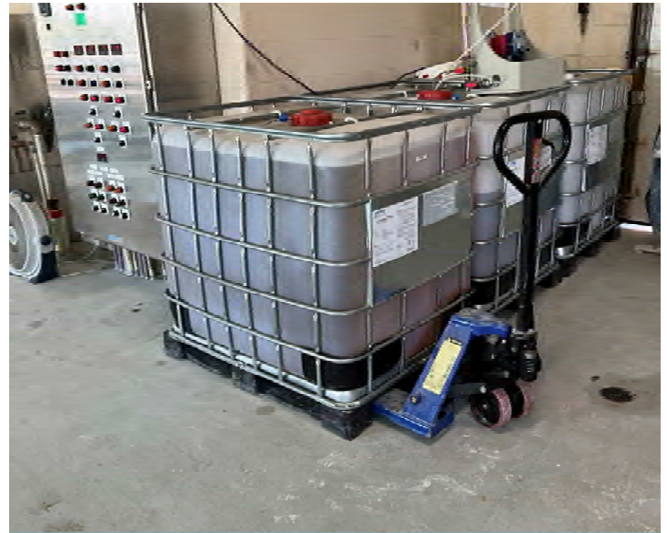
LimeCure25 storage totes and feed equipment
