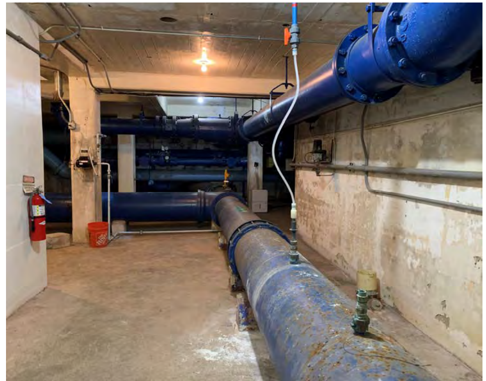
Filter effluent piping replacement
