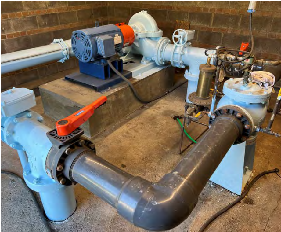
Gute Hill Booster Pump and Altitude Valve
