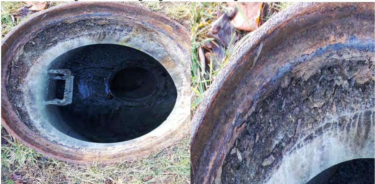
Figure 4 – MH Casting along Hintz Road – Discharge from PS-6 Force Main
