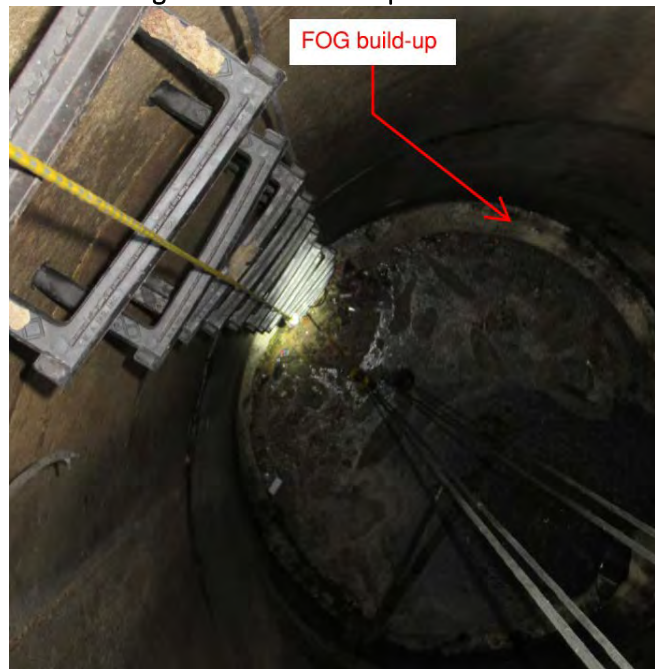
Figure 3 – FOG Buildup in Wet Well
