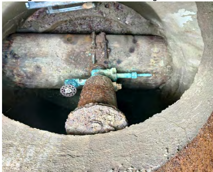
Figure 5 – Air relief on force main along Hintz Road
