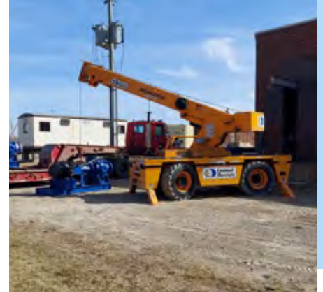
One of two new backwash pumps that were being unloaded for installation.
