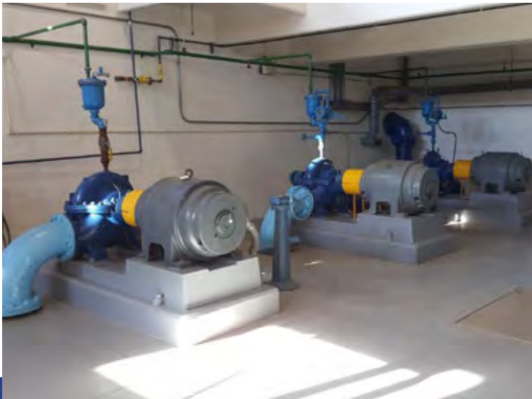
High Service Pumps 1, 2 and 3 shown above, pump 1 (furthest away) is being rebuilt.
