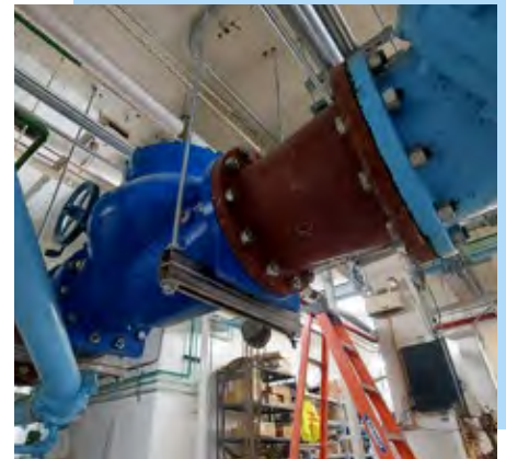
This pressure reducing valve (PRV) now safely controls the water pressure used during a filter backwash. This system backs up the two new backwash pumps.
