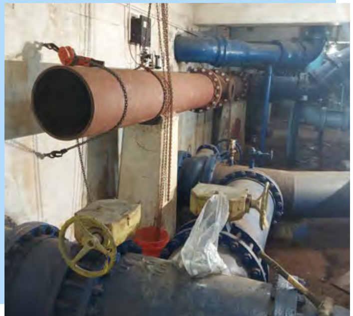
New 16" piping being installed in the subbasement of the Plant replacing a 80+ year old pipe that was ready to burst.
