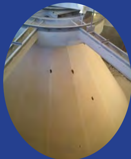
One of two Clarifiers at the Water Filtration Plant, the main bearing which required replacement, is located at the top of the cone which is 30 ft. deep.
