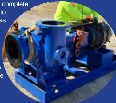
This is one of two new backwash pumps in service as of June 2021.
