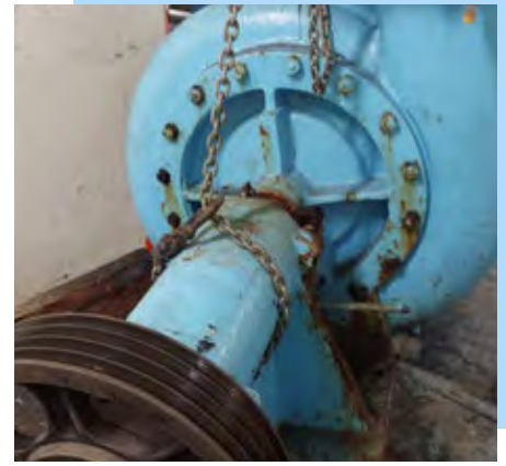
This original backwash pump was in service for 80+ years. There was no backup pump or usable backwash method if this failed.
