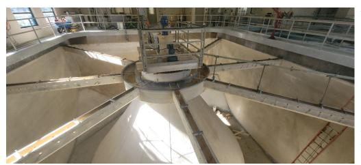
This is a photo of the South Clarifier. It shows we have removed all 286,000 gallons of water and are repairing and servicing the unit. This Clarifier is almost 30 ft. deep. Cleaning and inspections have to be done every 6 months. Parts have to be replaced regularly and paint touchups are constantly applied to surfaces that begin to rust.
