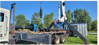
This well, located at the Water Filtration Plant has been tested and inspected. It needed some new components and other components were able to be made like new again. The well pipe and screen needed pressure and chemical cleaning. The photo shows the reinstallation of the well. This type of contract work is necessary every 6 to 8 years at a cost upwards of \$45,000.00.
