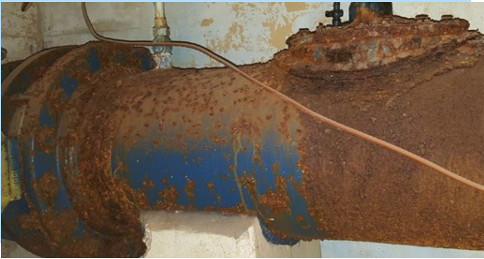
A portion of the old pipe was replaced.
