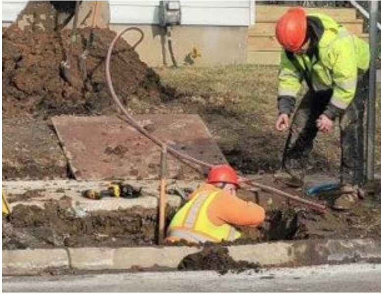
Lead service line being replaced at a residence
