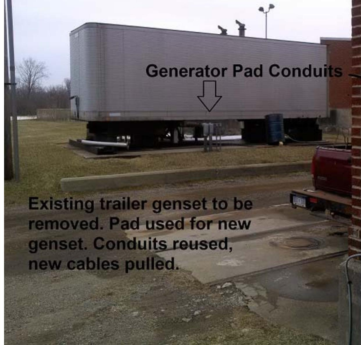
Existing trailer genset to be removed. Pad used for new genset. Conduits reused, new cables pulled.
