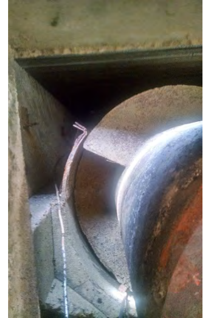
Worn channel and flights results in significant gaps between the flights and the channel
