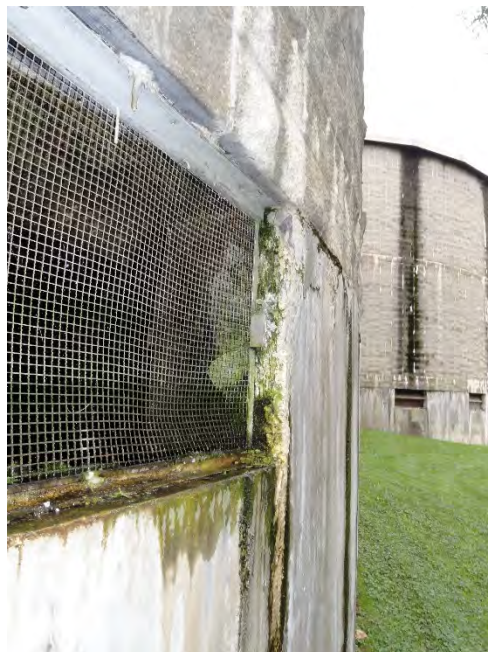
Picture 5. Nitrification Tower Structural Damage and Mold
