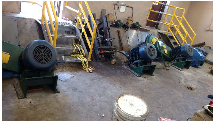
Picture 3. Screw Pump Motors
