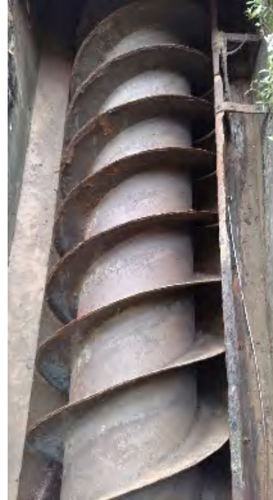
Existing screw pump.
