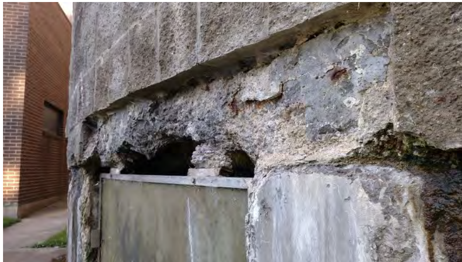
Picture 4. Nitrification Tower Structural Damage
