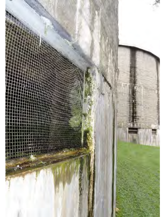
Towers damage from age and environment
