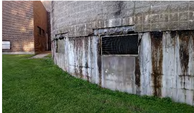
Tower structural damage
