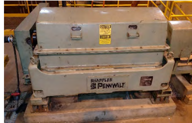
Existing solids centrifuge
