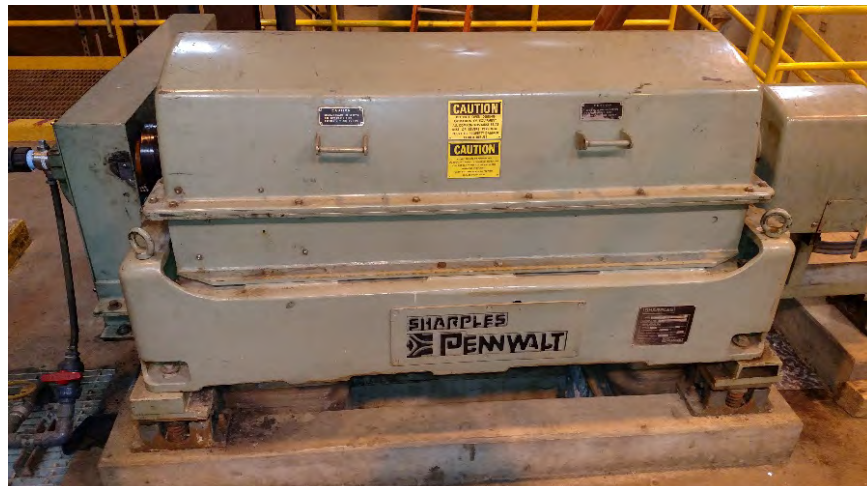
Picture 7. Solids Centrifuge (Front)
