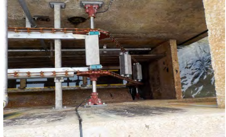
Example of Grit Tank System
