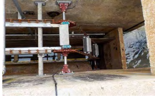
Example of Grit Tank System
