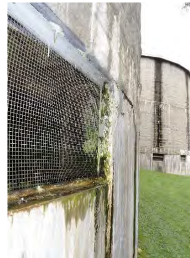
Towers damage from age and environment
