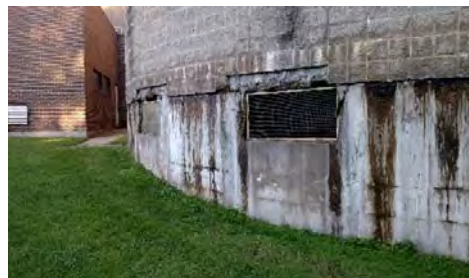
Tower structural damage
