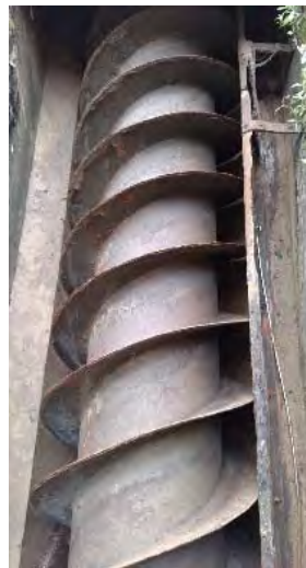
Existing screw pump.
