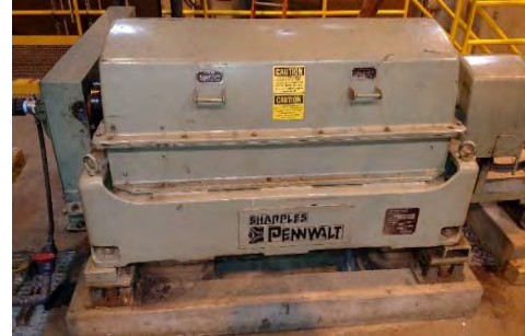
Existing solids centrifuge
