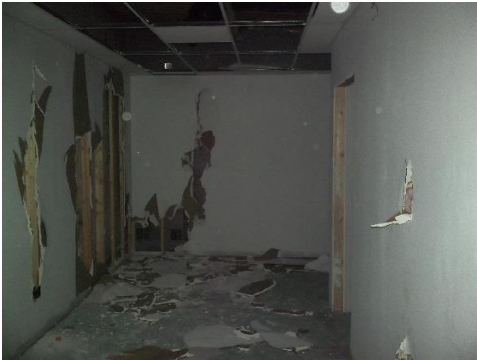
Interior view of 910 East Main Street
