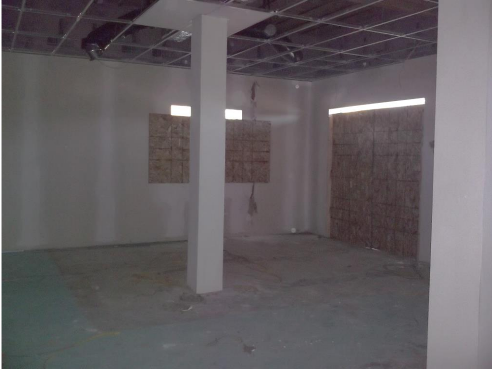
Interior view of 910 East Main Street
