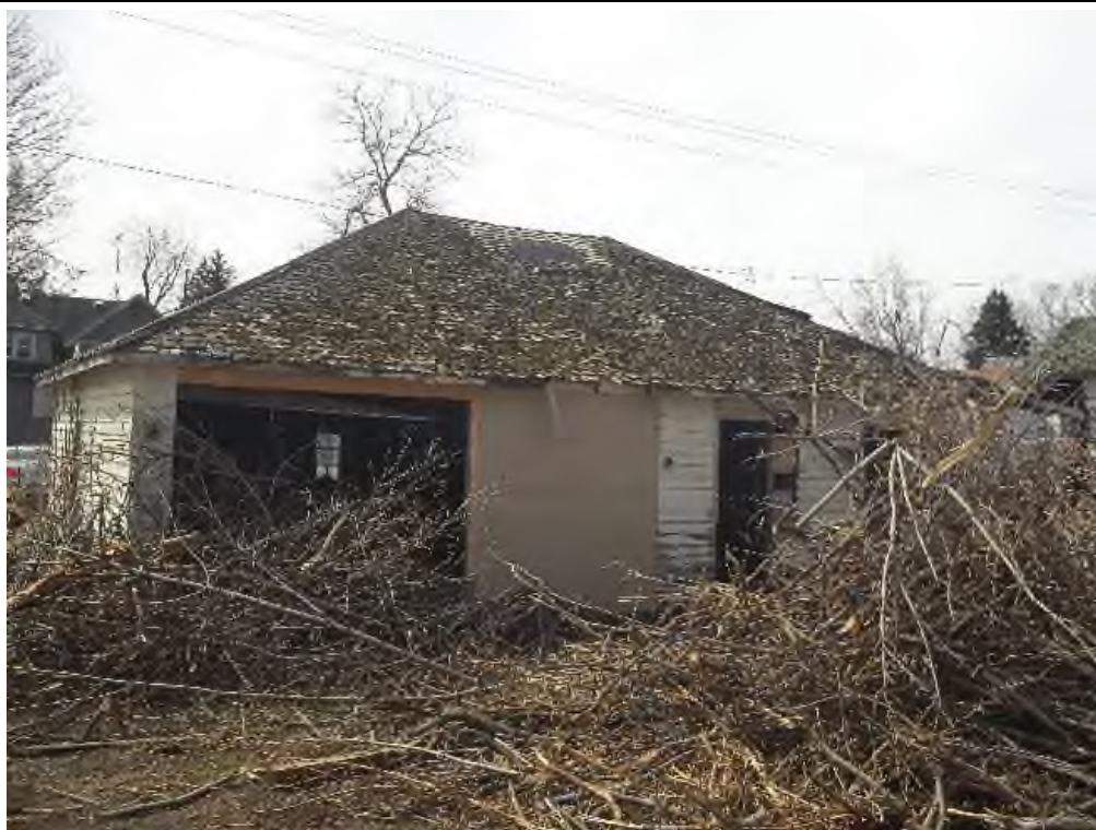
View of detached garage associated with 834 E. Main Street
