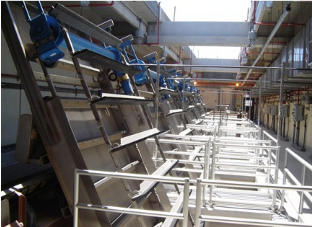
Picture may not reflect this specific project
