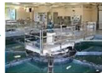
Calcium Hydroxide is fed into processing units called "Clarifiers". When the solids contact Clarifiers, raw water mixes with the calcium hydroxide to remove hardness. During 2016 the lime softening process reduced hardness by 59%
